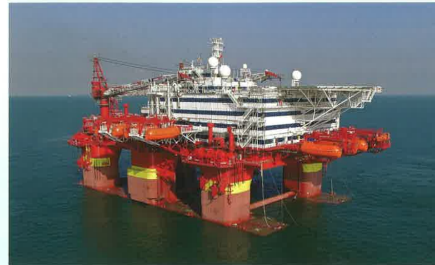
Keppel FELS has delivered Floatel Triumph , a fifth high-specification accommodation semi-submersible built to Keppel's proprietary SSAU™5000NG design, safely and on time.
