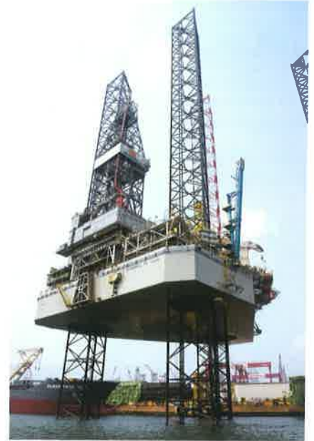
ARABDRILL 70 is the fourth KFELS B Class jackup rig to work for Arabian Drilling Company. It was completed three days ahead of schedule, on budget and with a perfect safety record.
