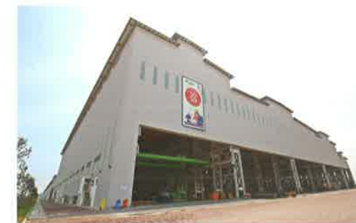
Sembcorp Marine's new steel structure fabrication workshop is expected to boost its steel fabrication capacity in Southeast Asia.
