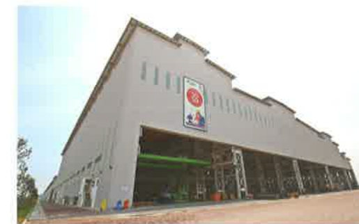
Sembcorp Marine's new steel structure fabrication workshop is expected to boost its steel fabrication capacity in Southeast Asia.
