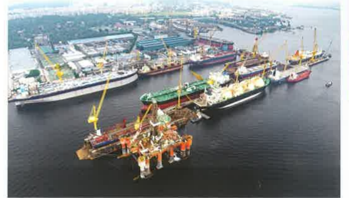
Aerial view of Sembcorp Marine Admiralty Yard, showing concurrent repair of two LNG vessels.
