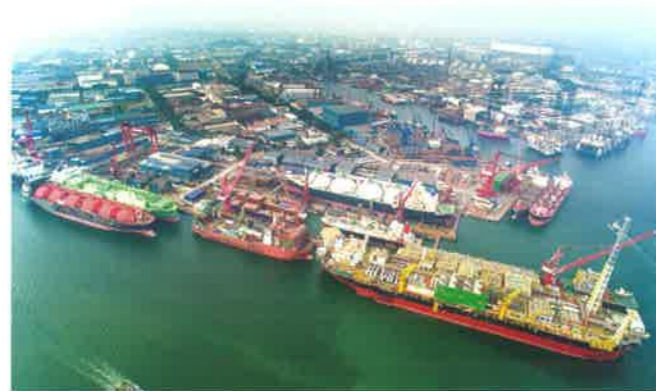
FPSO vessel Cidade de Caraguatatuba MV27 currently undergoing module integration work in Keppel Shipyard.
