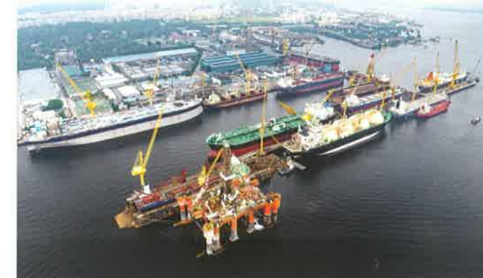
Aerial view of Sembcorp Marine Admiralty Yard, showing concurrent repair of two LNG vessels.
