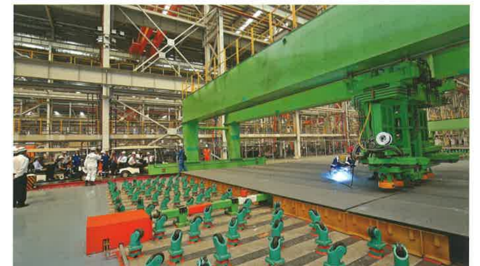
The 120,000-sqm facility included a fully-automated panel production line that delivers high quality welding precision and efficiency.
