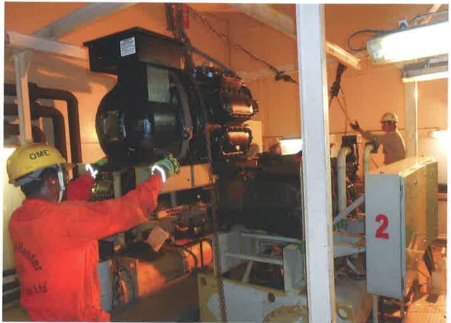
HVAC - Installation of semi-hermetic compressor.
