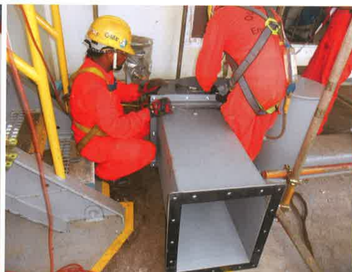
Ducting - Installation of ducting.
