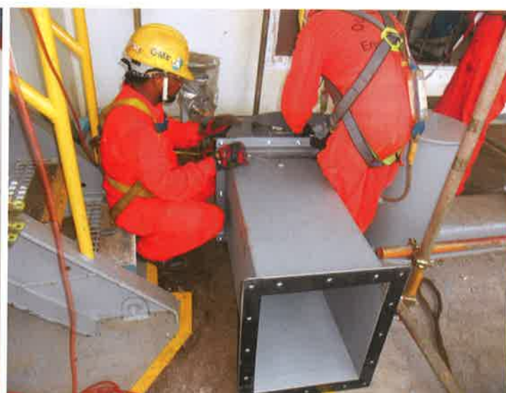
Ducting - Installation of ducting.
