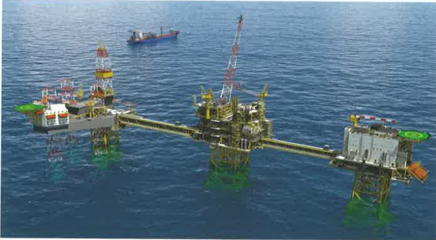
The EPC contract from Maersk Oil North Sea includes the building of the Central Processing Facility plus two connecting bridges, Wellhead Platform and Utilities and Living Quarters Platform Topsides for the Culzean Field Development.
