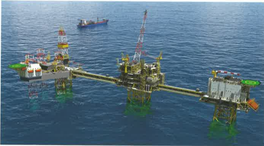
The EPC contract from Maersk Oil North Sea includes the building of the Central Processing Facility plus two connecting bridges, Wellhead Platform and Utilities and Living Quarters Platform Topsides for the Culzean Field Development.
