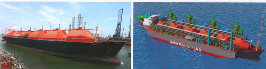
Keppel Shipyard is currently performing the conversion of another existing Moss type Liquefied Natural Gas (LNG) carrier, the HILLI (left), into a Golar Floating Liquefaction (GoFLNG) facility (right).
