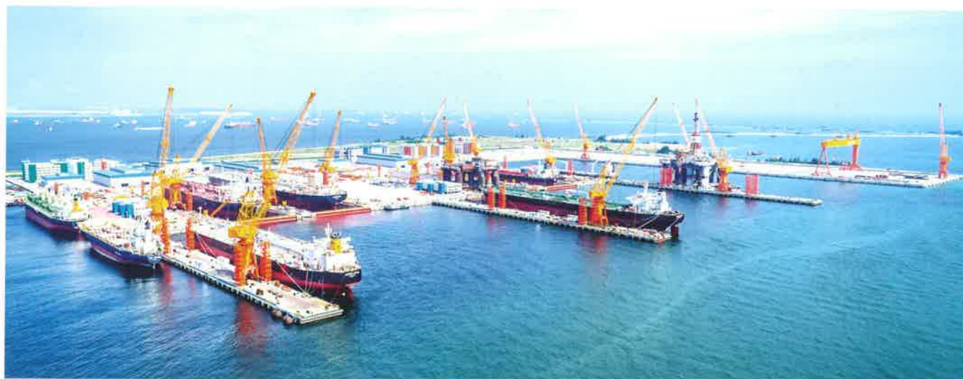
Sembcorp Marine's new yard facility - Sembmarine Integrated Yard @ Tuas.
