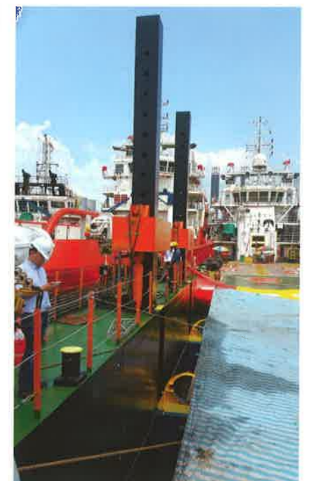
Barge Conversion to Floating Dock.
