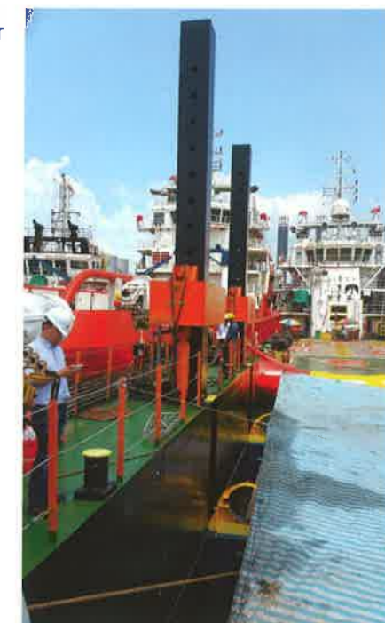
Barge Conversion to Floating Dock.
