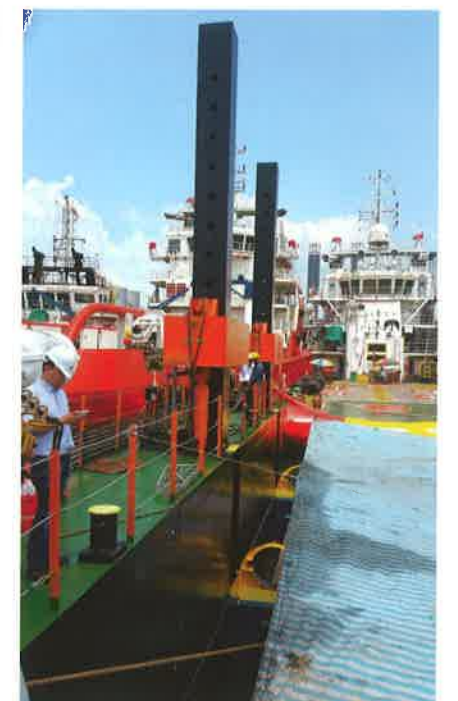
Barge Conversion to Floating Dock.
