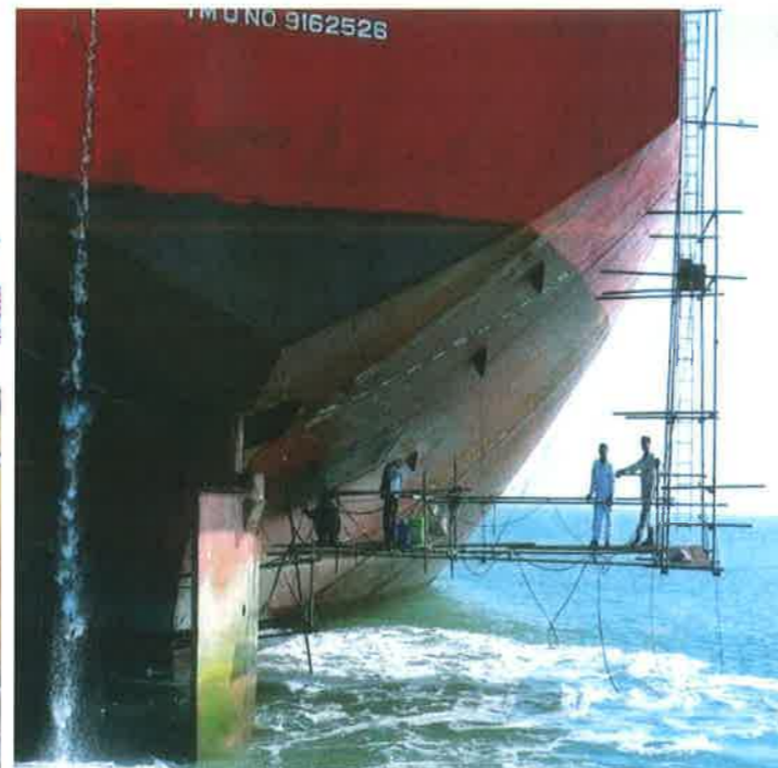
Side shell repair with handing staging at anchorage.
