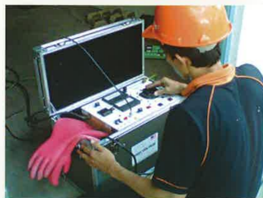
Hi-Pot testing in progress.
