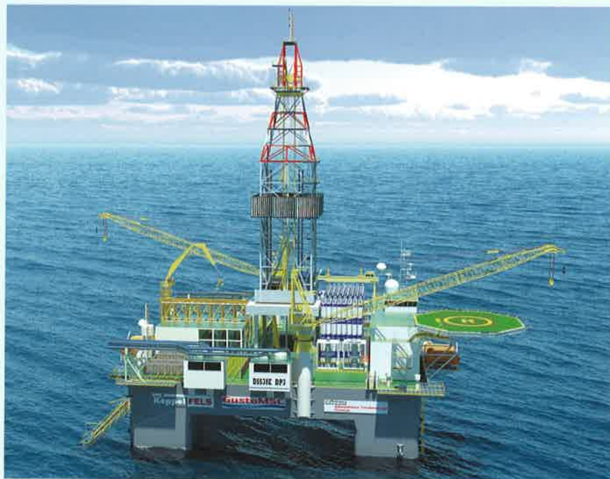
Keppel will be building a total of six DSS™ 38E semis for Sete Brasil.
