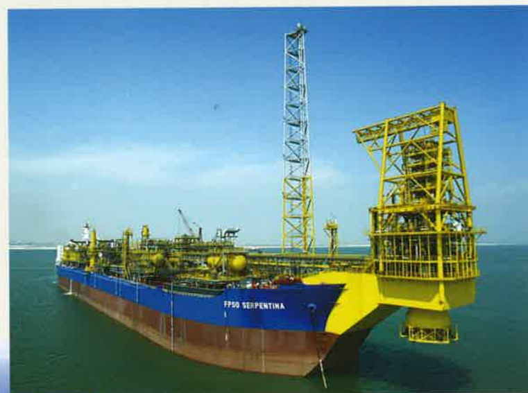
Harris Pye Singapore has carried out many repairs on FPSO Serpentina, from boiler retubing to heavy fuel oil modifications. (Photo courtesy of SBM)
