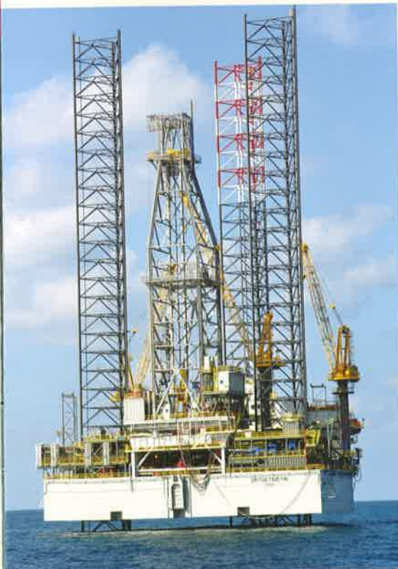
Excel Marco provides turnkey integrated vessel/marine management, telecommunication, safety systems on the first new-built Super M2 Jack-up Drilling Rigs for Maritime Industrial Services, based in Sharjah.
